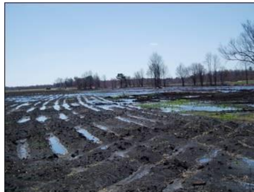
Figure 25: Restoration activities to reduce soil compaction can include disking in a cross-disk pattern.
